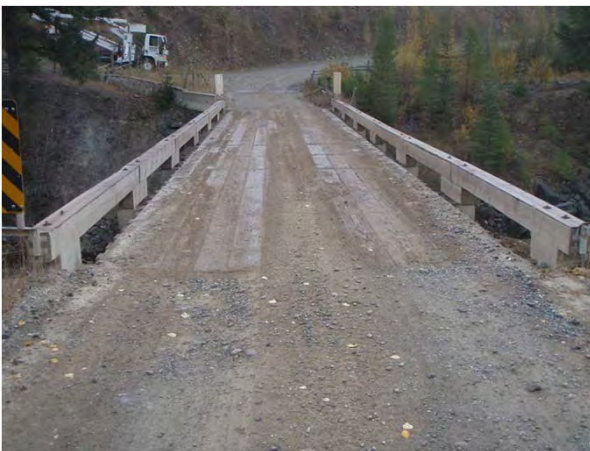
Figure 1-5: Looking towards camp end.
