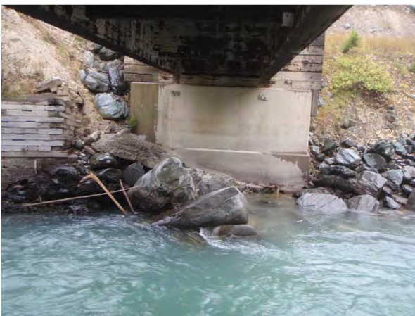
Figure 1-11: Camp end abutment.
