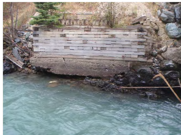
Figure 1-12: Old bridge abutment upstream of camp end abutment.
