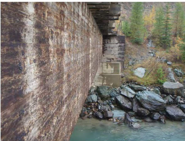
Figure 1-9: Upstream face of girder 1.
