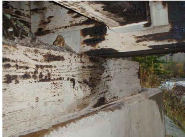
Figure 1-14: Woods end cap beam.
