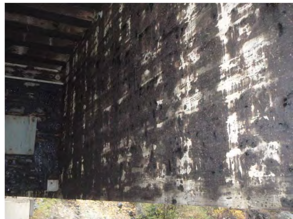
Figure 1-10: Typical interior face of girders.
