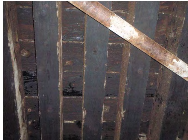
Figure 1-8: Typical underside of deck.
