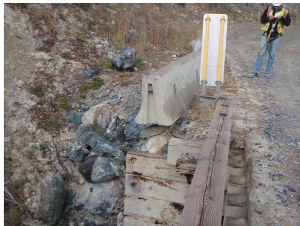
Figure 1-6: Camp end upstream concrete barrier.
