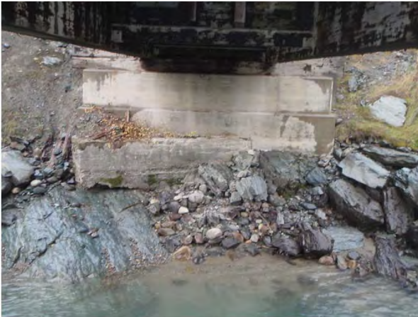
Figure 1-13: Woods end abutment.
