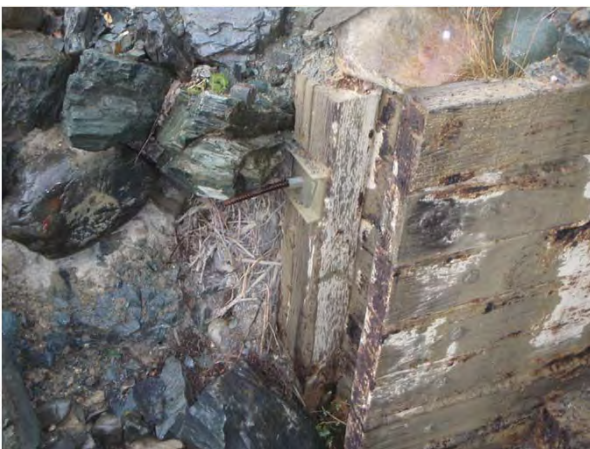
Figure 1-17: Typical wing wall.
